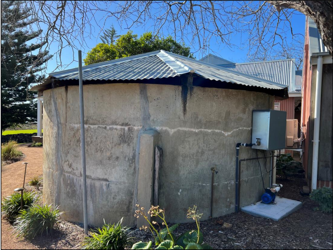
Site Photograph 6.7.1 Aboveground storage tank observed adjacent the sheet metal residences, viewed facing north-west.
