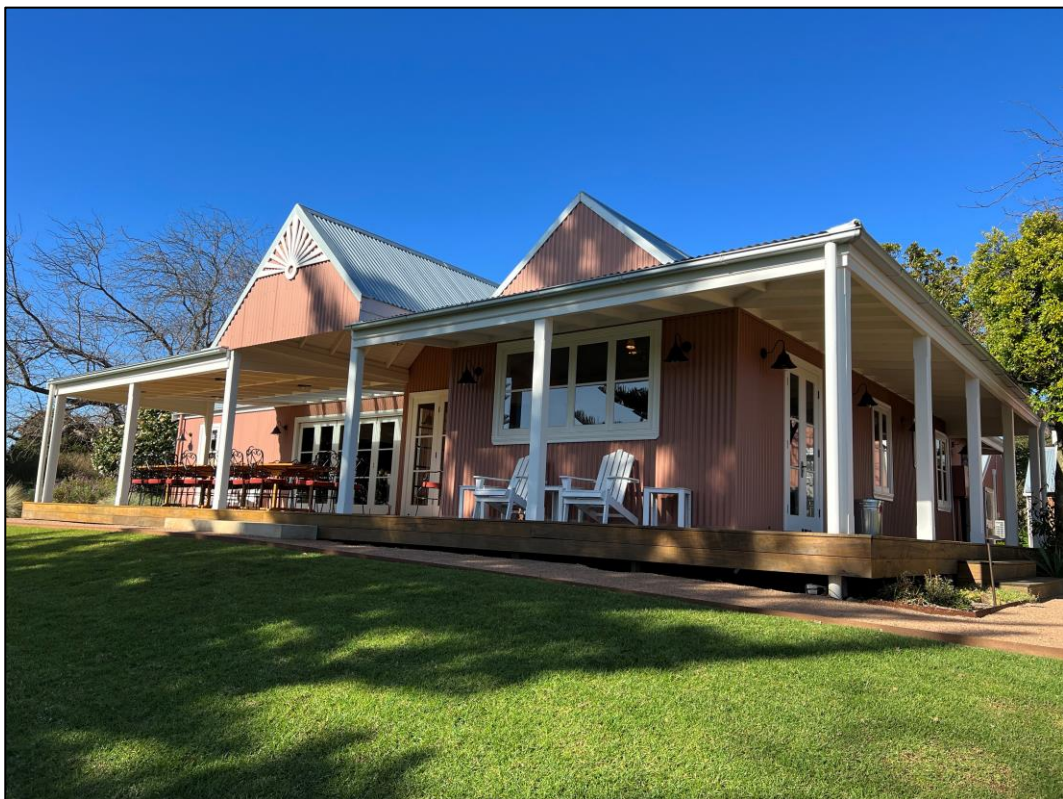
Site Photograph 6.2.6 Sheet metal residential structure located within the southern portion of the site, viewed facing south-east.
