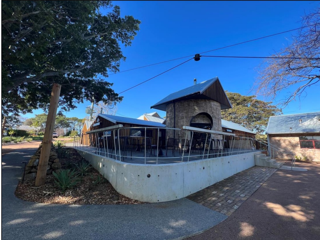
Site Photograph 6.2.5 Timber and concrete venue room located on the southern boundary of the site, viewed facing southeast.
