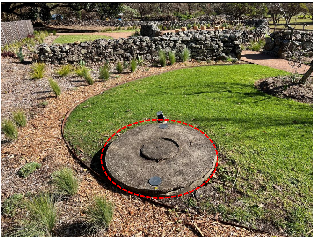
Site Photograph 6.7.4 Underground septic tank, located on the northern boundary of the pool, viewed facing west.
